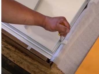
Now lift the headwall out of the carton, and place it in position. With the headwall top tilted back against the building wall and the bottom away, pass the medical gas piping through the appropriate hole in the ceiling mounting plate. Push the headwall up and flat against the building wall, lift it up against the ceiling mounting plate and fasten the headwall to the blocking that was placed within the building wall.
